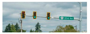
Safety improvements include installing reflective backplates for traffic signal heads.
